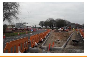
Topsoil has been removed and stored for reuse from the inner island of Farmers Roundabout. This was undertaken to facilitate traffic signal system duct laying and full depth carriageway construction in the coming months which will create the new road widening areas and allow for the signalisation works that are being brought forward as part of the Farmers Roundabout Improvement Scheme.
